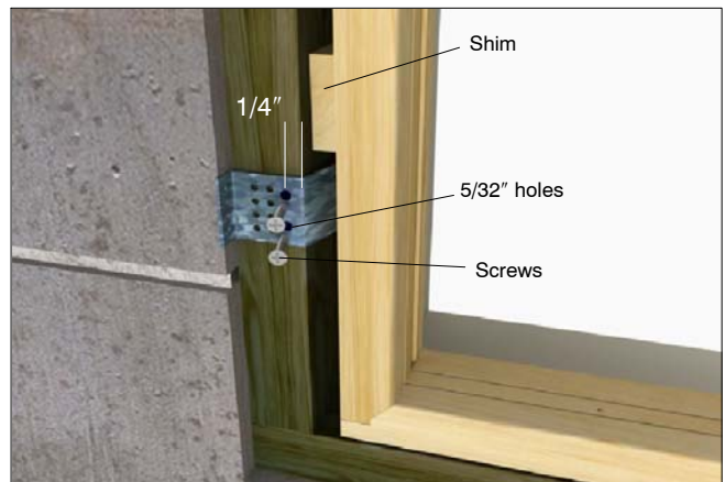
Figure 8: Attaching window with masonry clips or installation brackets.
